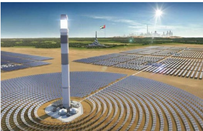
Mohammed bin Rashid Al Maktoum Solar Park
