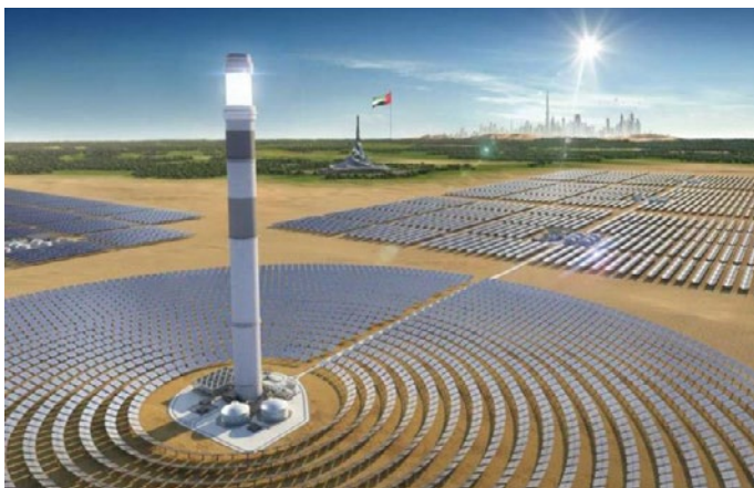
Mohammed bin Rashid Al Maktoum Solar Park
